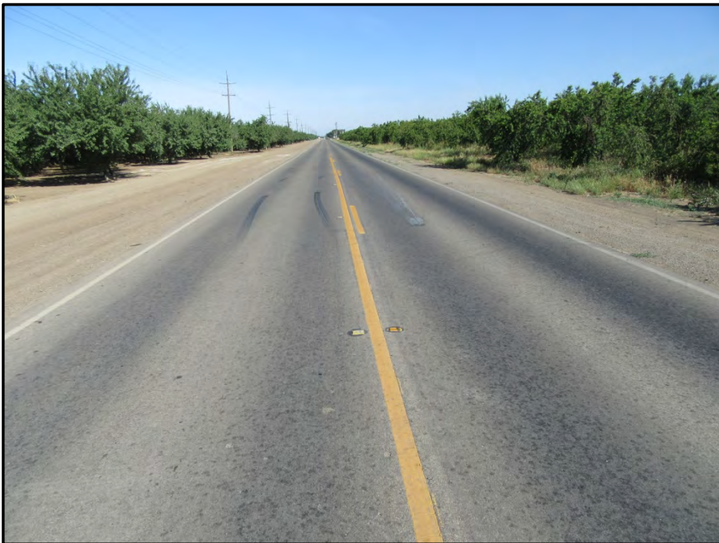
River Road, just northwest of the community of Grayson, looking northwest; 05/30/17. The new pipeline will be constructed either in the road or along one of the road shoulders.
