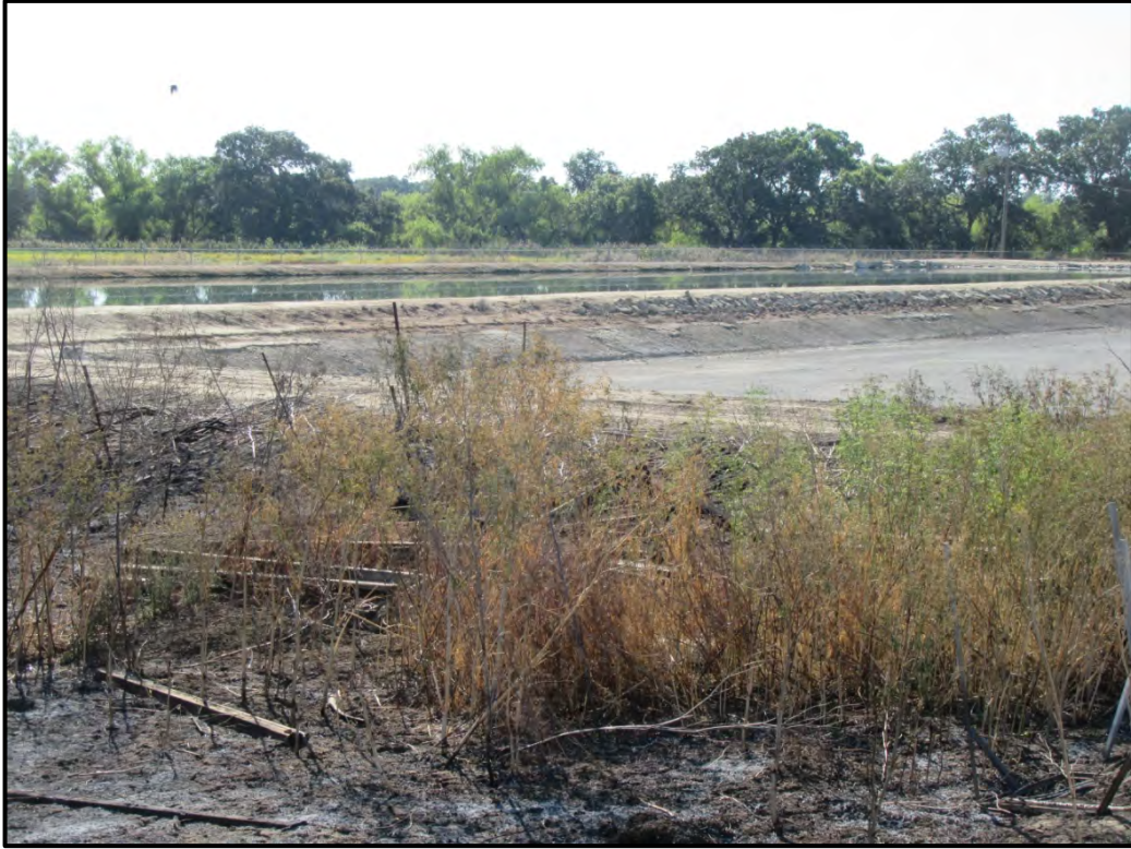
Grayson WWTP Ponds, looking east toward the San Joaquin River corridor; 05/30/17.
