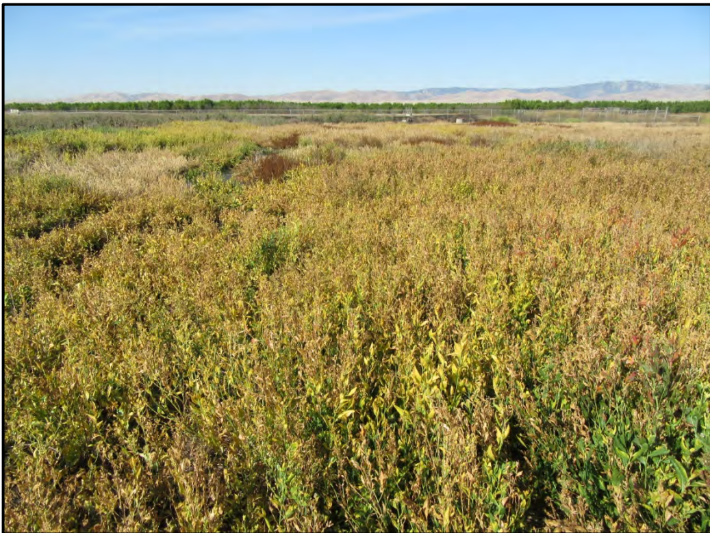
Existing disposal area in the Grayson WWTP, looking southwest toward the ponds; 05/30/17.
