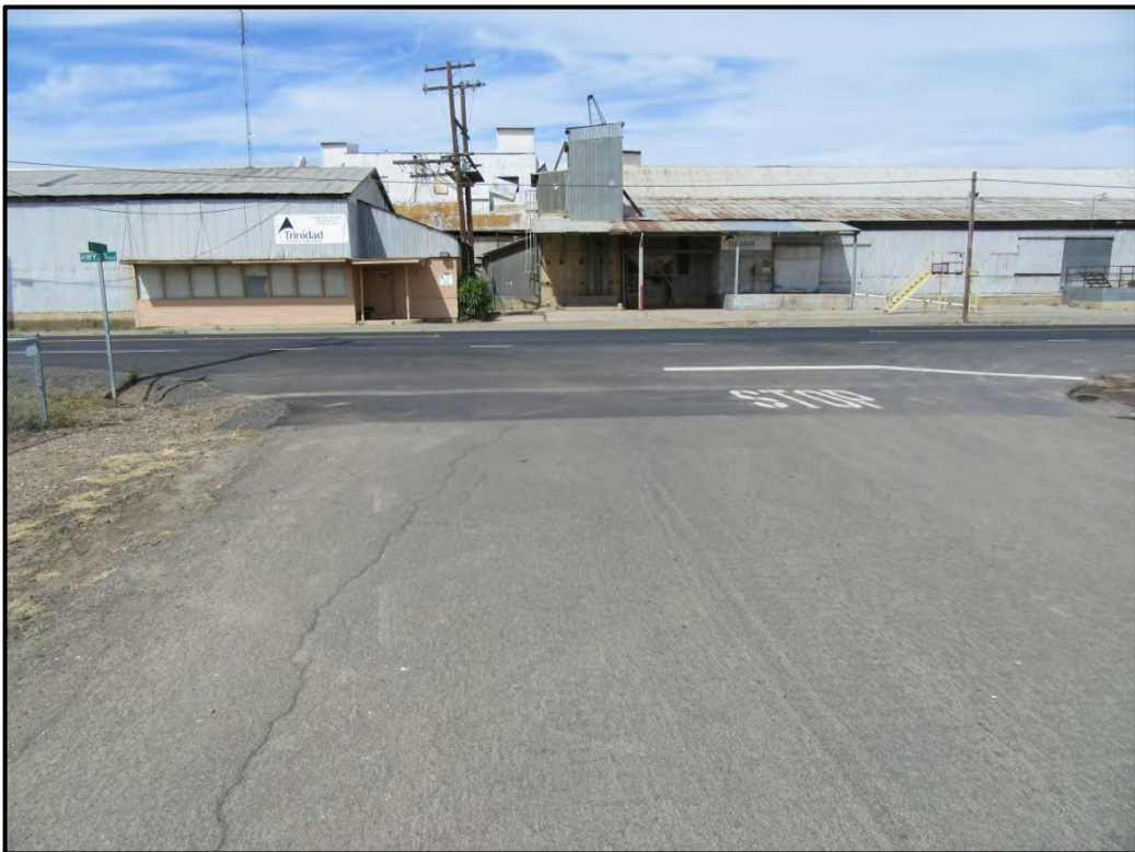
B Street in the community of Westley looking northeast; 05/30/17. Construction of the pipeline along this alignment would involve a bore & jack under this building and the railroad tracks.
