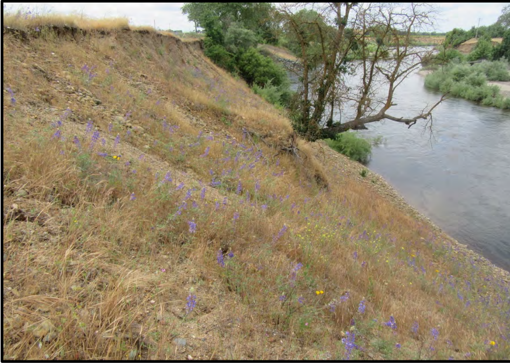
Meiss Road Upstream, looking west at the eroded slope; 05/17/19.
