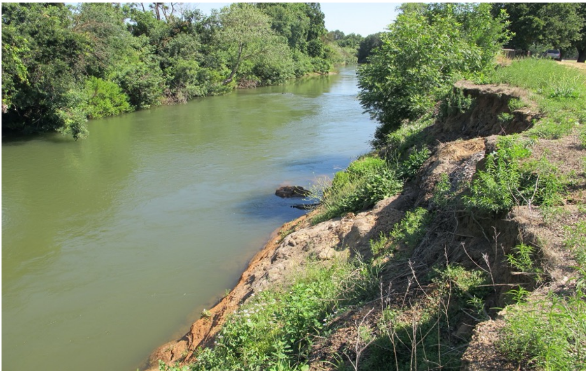
Figure 8-A. Looking upstream from the Cosumnes Road Upstream site. Clear evidence of significant erosion at the top of the levee. Little substantial vegetation on the levee's slope to help mitigate erosive forces during extreme flow events.
