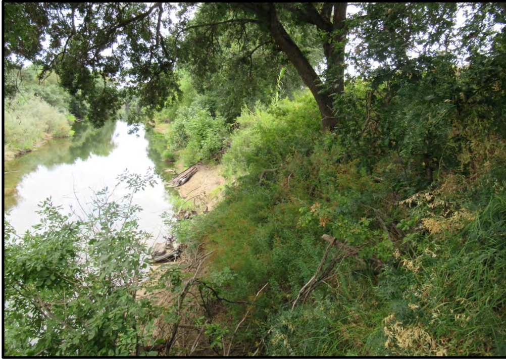
Mile Marker 19, looking southwest from the east end of the repair site; 08/05/19.
