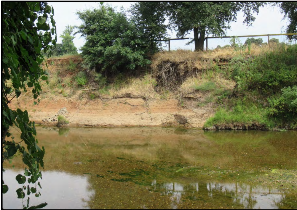
Cosumnes Road Upstream, looking southeast at the eroded levee slope from across the river; 08/05/19.
