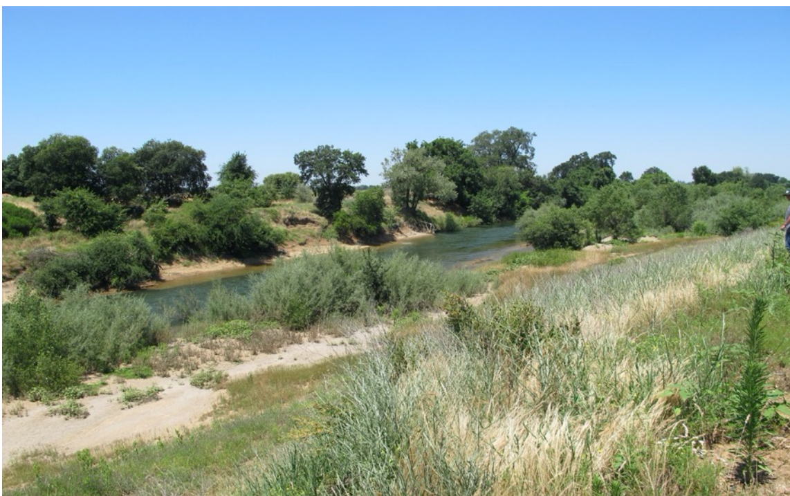
Figure 4-A. Photo from levee at Keating Road site. Significant erosion at levee toe had led to the formation of sandy substrates in “upland” area. Vegetation along both banks consists primarily of shrubs and willows offering little shaded riparian area.
