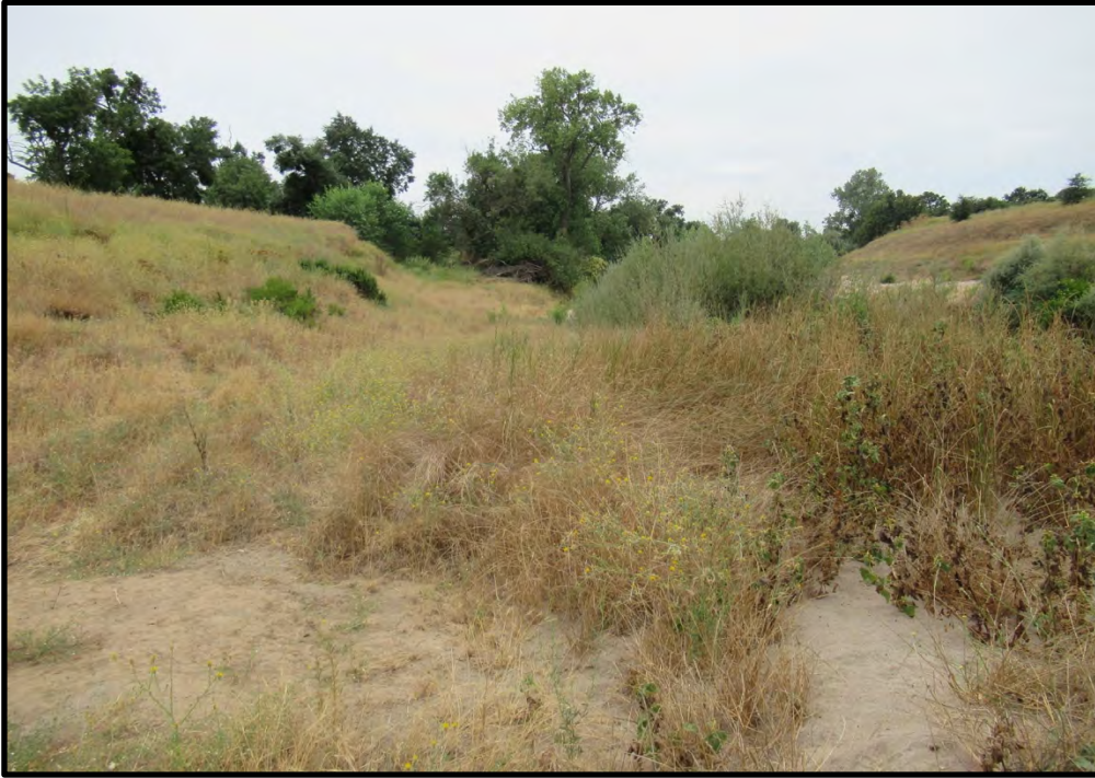
Keating Road site, looking south from the north end of the repair site; 08/05/19.
