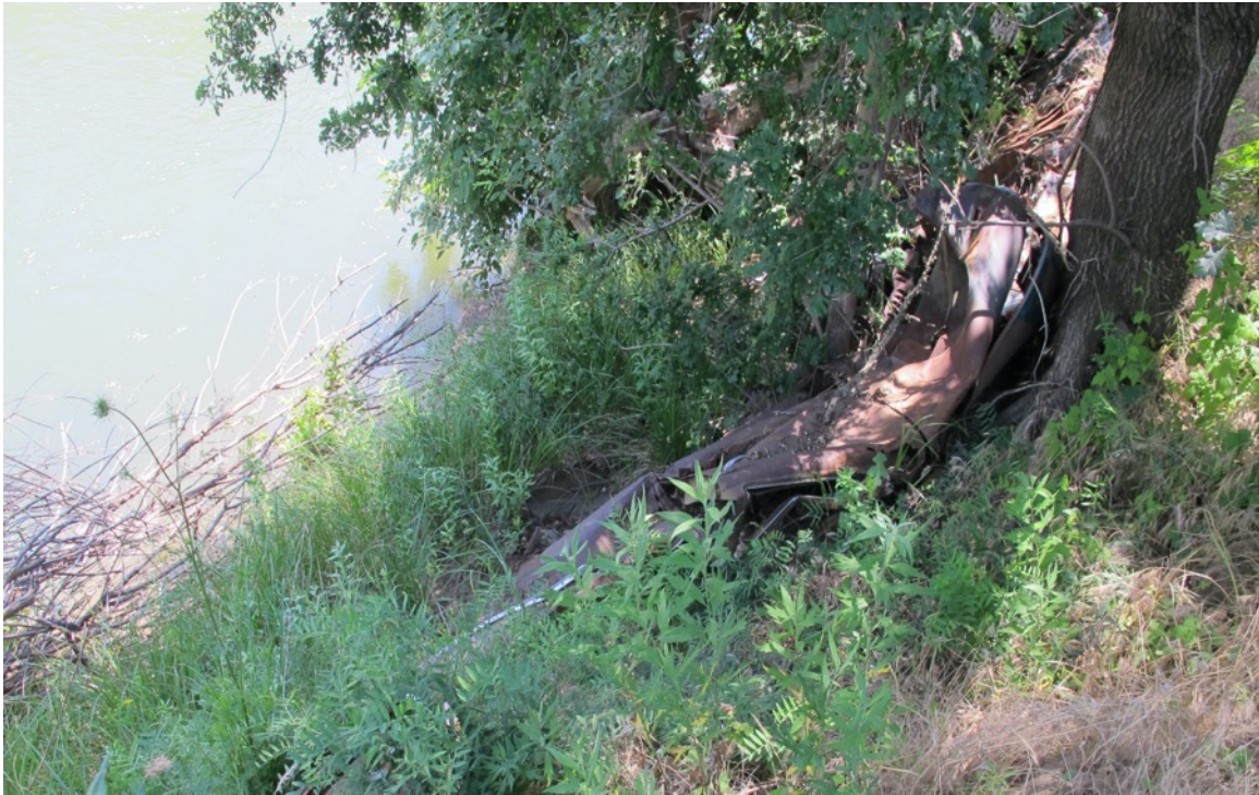
Figure 7-A. Several compacted cars lined the bank at the Mile Marker 19 site. Most likely placed as erosion control in a previous era.
