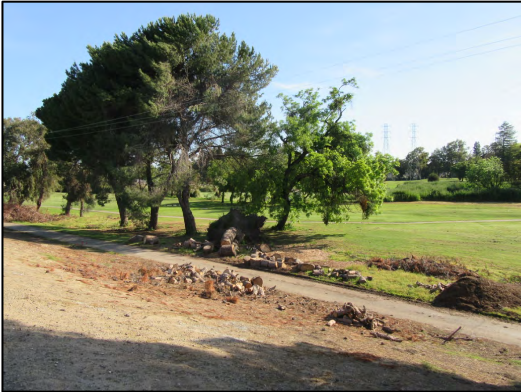
Trees in the golf course adjacent to the levee that have died, looking northeast from Station 48+50; 04/21/17. Saturated soil from seepage likely contributed to these trees dying.
