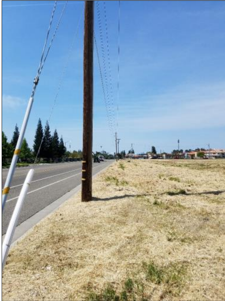
Figure 3 Utility pole along southeast edge of project area, facing west.
