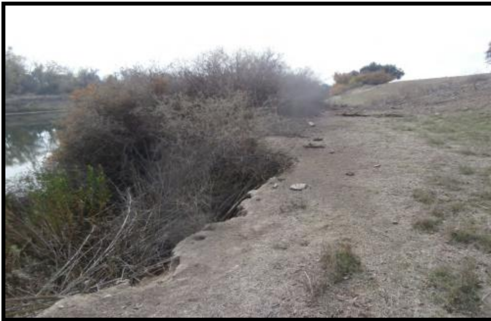
Photo 2-1 Mass wasting at project site. Levee visible in upper right corner.
